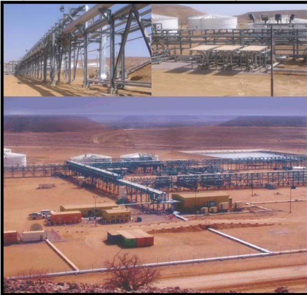
FEED & Detailed Engineering - Onshore Processing Facility – Block 51 BAK Processing Facilities, Yemen
