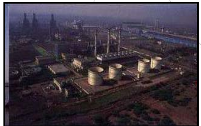
De-Bottlenecking Study of Process Facilities & SBHT Lines - Hazira Plant (India) for ONGC
