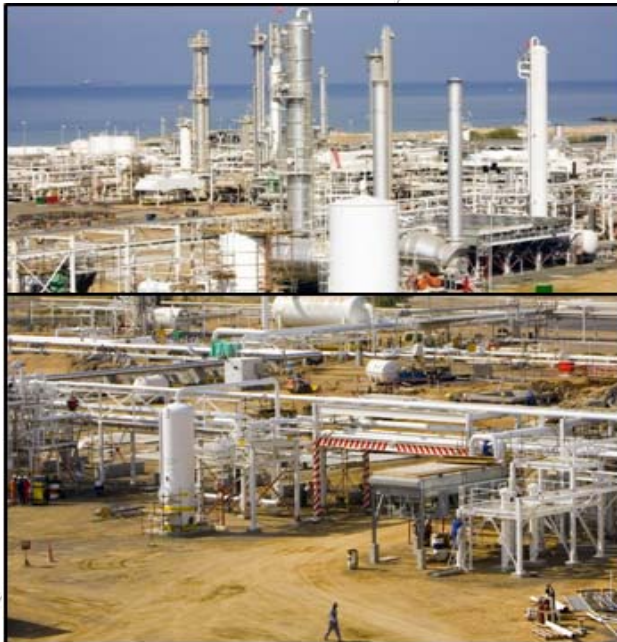
FEED & Detail Engineering - Saleh Phase 1 & 2 Facility Modification, Ras Al Khaimah
